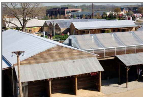
Terrain at Styers - 914 Baltimore Pike Glen Mills, PA
